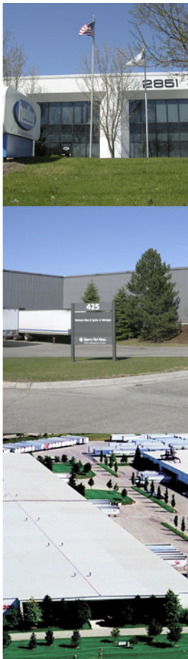
A sample of some of the many buildings included in CORE's latest acquisition, West Michigan Industrial.
